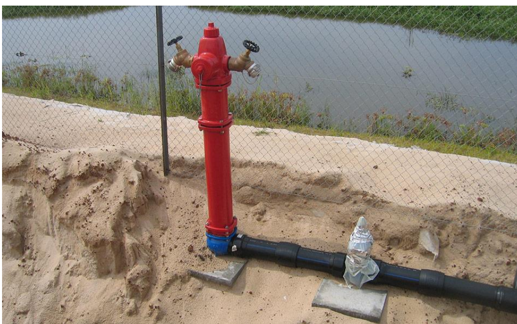
Figure 3.9. Hydrant installation with an insulated gate valve
