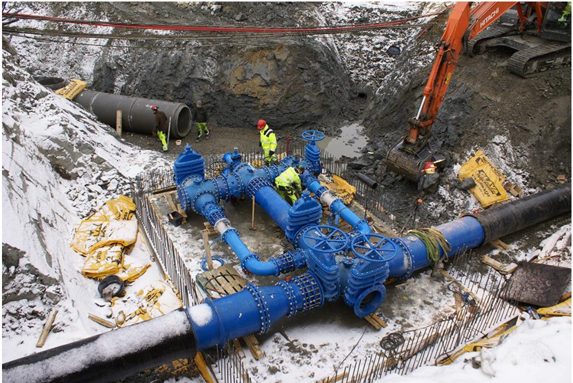
Figure 6.1. Installation of valves in cold climate
