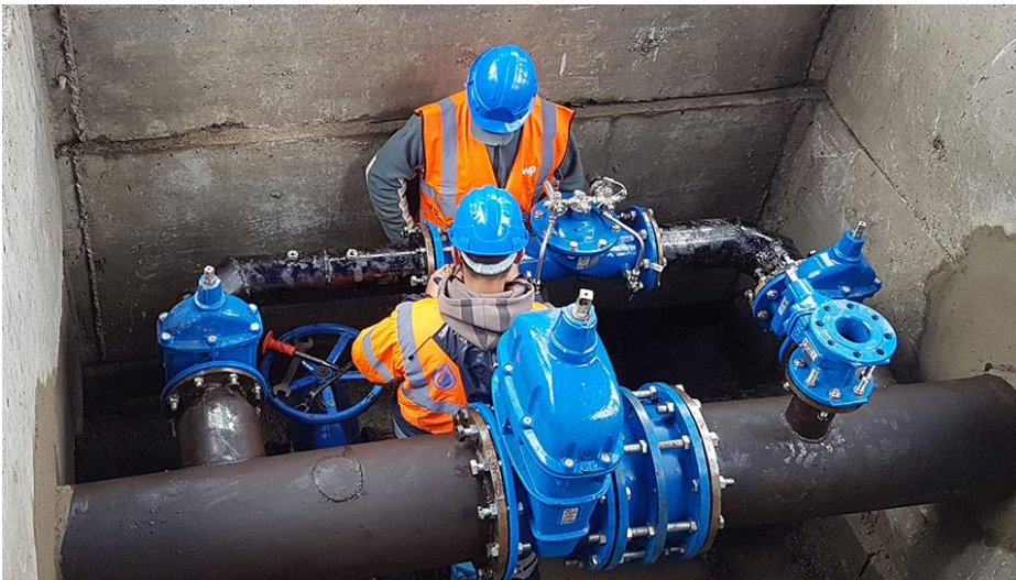
Figure 5.3. Installation with gate valves and control valve
